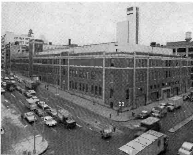
The CBS Broadcast Center, at the corner of Manhattan's West 57th Street and 11th Avenue, includes six television studios surrounded by technical equipment and supporting facilities in its three buildings.
