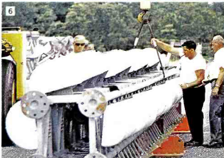
(6) The complex horizontal pattern of this UHF Panel antenna was tailored to avoid signal reflections from a mountain at the rear of the transmitting site, while meeting specific pattern requirements in three other directions. Each Zee-Panel radiating element is fully protected by its radome cover.
