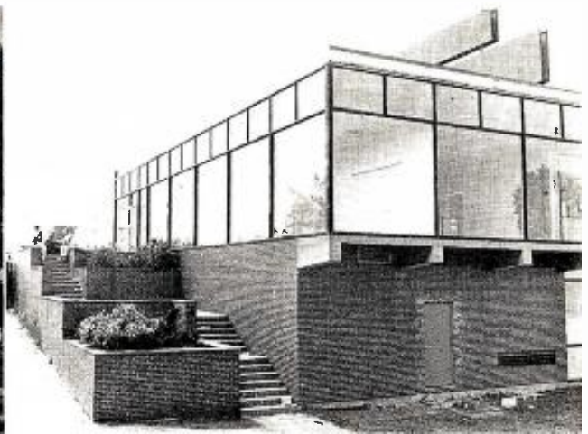
at 50 Morrissey Boulevard in Boston. BBI's WCVB-TV hopes to operate from its converted tractor plant in Needham should it win an eventual green light from the FCC.
