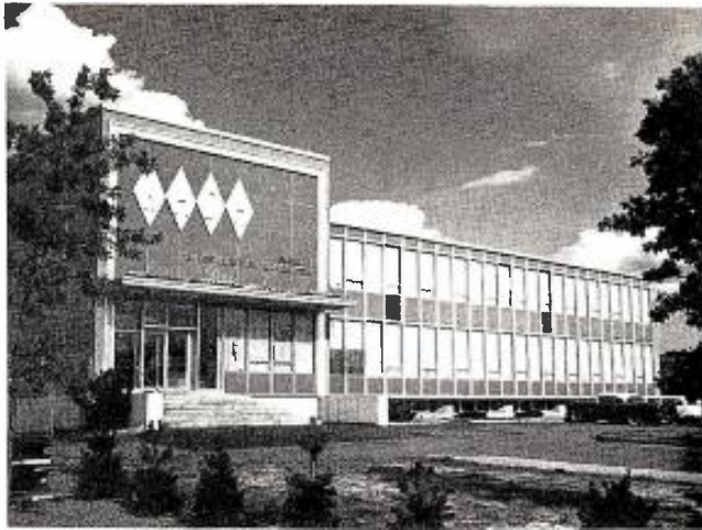
What is, what may be the structural envelope for channel 5. The Boston Herald-Traveler Corp.'s WHDH-TV has operated for 10 years from the broadcast plant pictured at left above,
