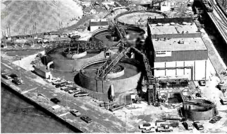
Republic's Steel Plant Water Treatment Plant, our latest addition, cleans and treats water used in the steelmaking process to tap water clarity. Cost: $8 million
