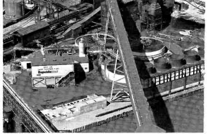
Republic's West Side Water Treatment Plant Original cost: $3 million Additional treatment facilities: $7 million
