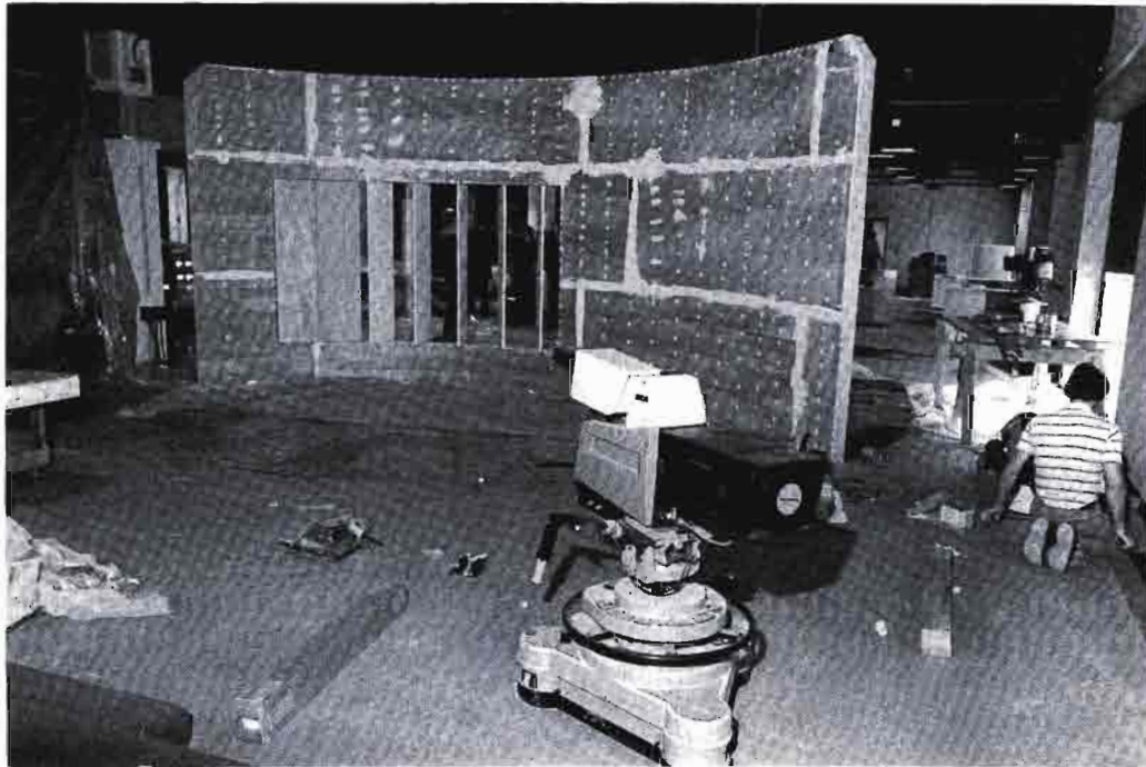
Centerpiece. Three of the nine sets in the Atlanta headquarters of the Cable News Network will be mounted on a turntable topped by a Y-shaped partition. One set will contain a one-man anchor desk; the other sets will be used for talk shows and intimate interviews. All will rotate before the cameras on command.
