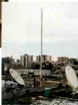
From downtown Denver, KMGH-TV broadcasts a low-power DTV signal using a Scala antenna mounted on its roof, and Larcam transmitter installed in the penthouse of its five-story building.
