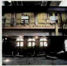
The building underwent extensive renovation.
