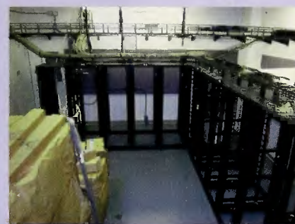
Let the wiring begin...
