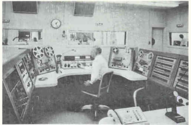
Master control serves five studios
