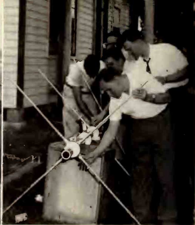
Assembling special airshipped antenna of KTHI-FM
