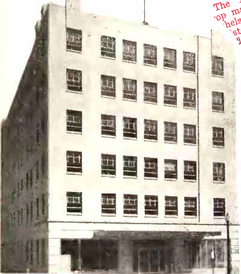
NEW GARLINGHOUSE BLDG.
