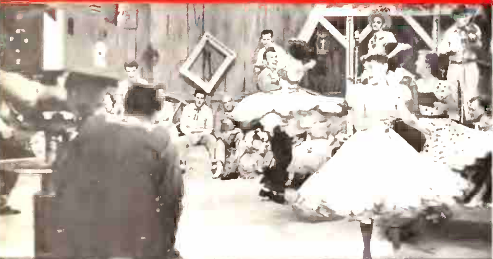
In a demonstration of ingenuity, typical of WKY-TV operation, an electric fork lift was employed to permit the rapid transition from low-angle to high-angle shots and the mobility necessary to follow the whirling pace of America's top square dance specialists.
