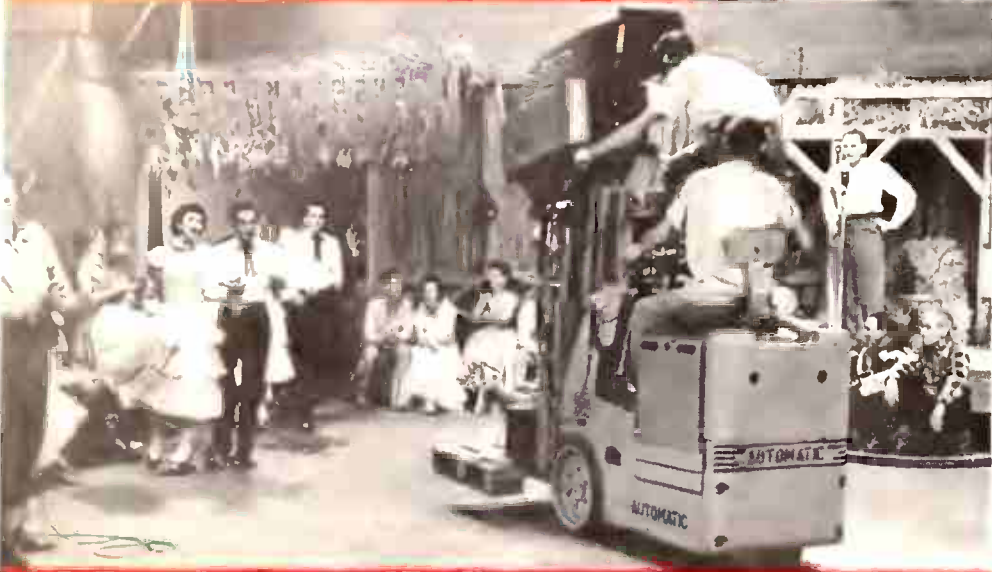
In a demonstration of ingenuity, typical of WKY-TV operation, an electric fork lift was employed to permit the rapid transition from low-angle to high-angle shots and the mobility necessary to follow the whirling pace of America's top square dance specialists.
