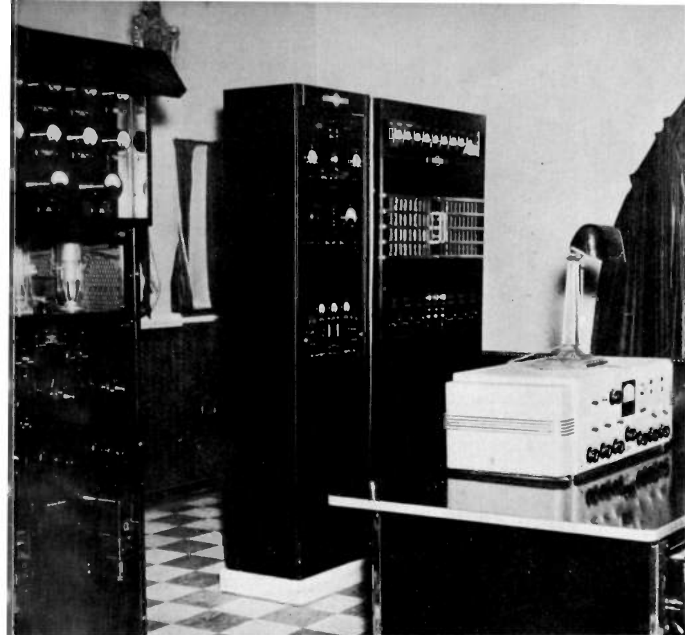
Inside the WOKO transmitter building on the opposite page, is the 1000 watt transmitter, itself. Through the facilities shown here you receive programs from WOKO from 7 a.m. until 2 a.m. on 1430 kilocycles.
