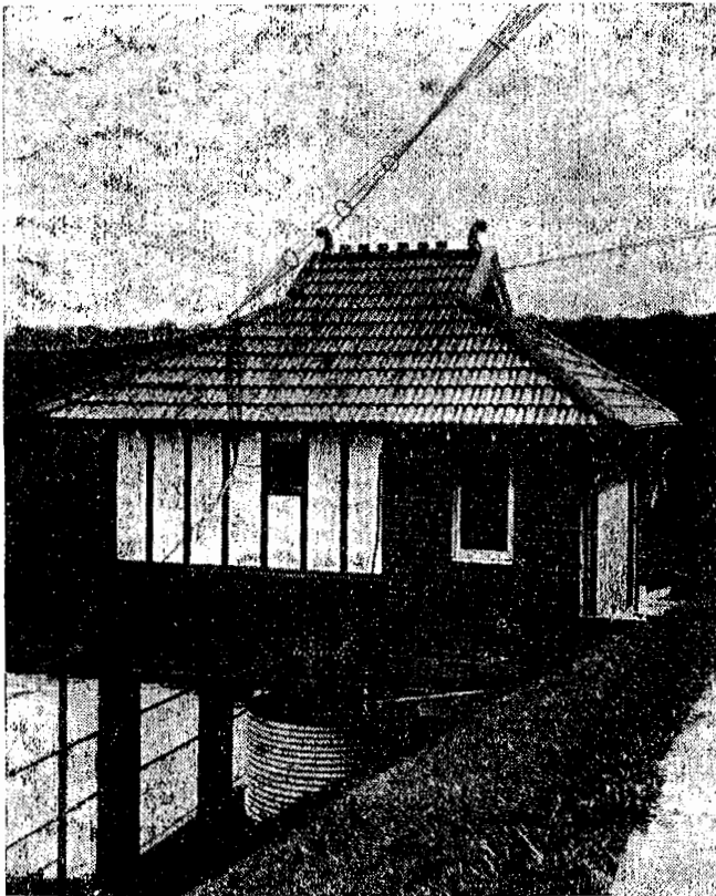
On August 23, 1926, the Theosophical Society's station 2GB began operating in Sydney. The original transmitter was housed in this small building in the grounds of Bishop Leadbeater's residence in Mosman, and at the time was the only broadcasting transmitter using a quartz crystal for frequency control.
