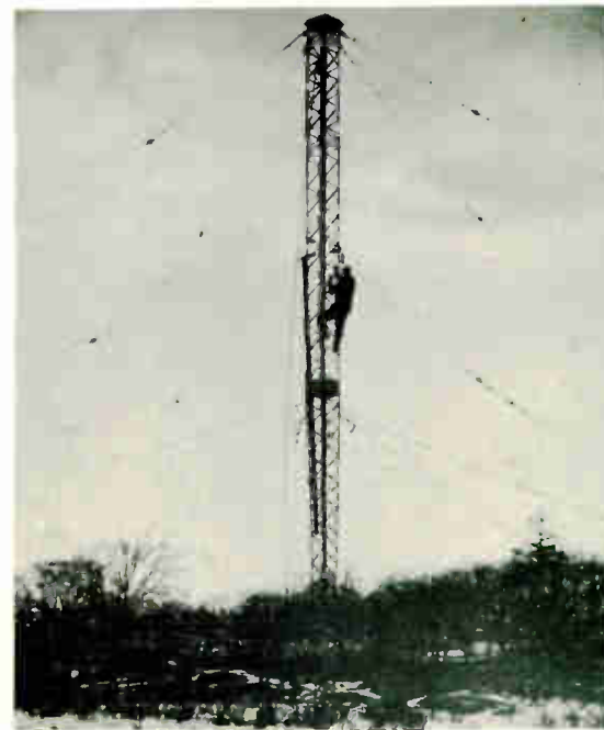
Transmitter Tower during construction — mid-winter 1949-1950
