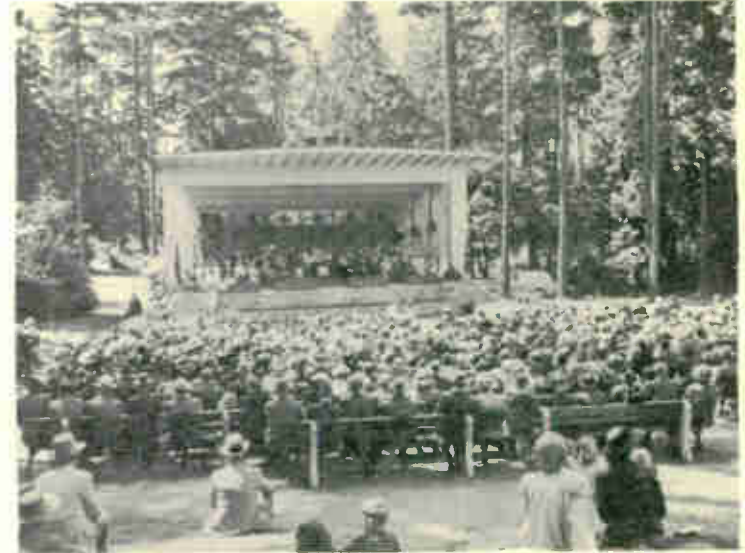
The New Band Shell at Beacon Hill Park
