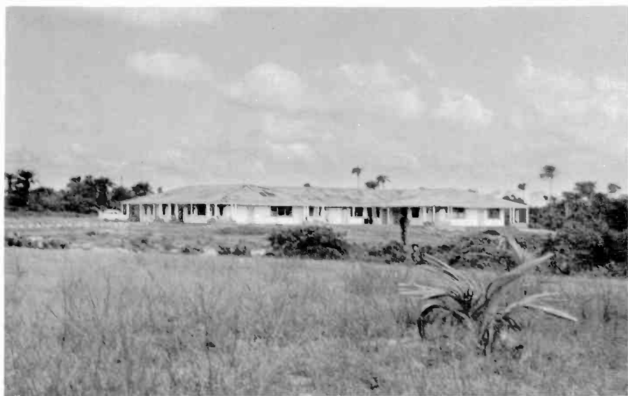
ELWA Hospital with car at main entrance.
