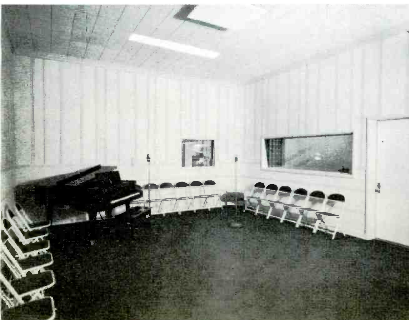
STUDIO A. This is the front of the studio with the long window opening into the lobby. Indirect lighting for reading ease is used throughout the studios. Treatment of walls and ceiling is in accordance with expert acoustical developments.
