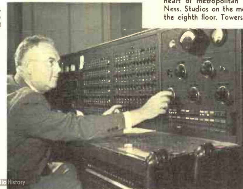
KFRC Master Control, Engineer Don Cameron—Where all KFRC studios, Don Lee Broadcasting System, Mutual Broadcasting System and overseas news operations and switching are performed.
