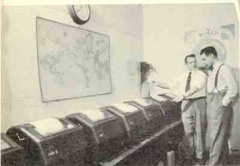
KFRC Teletype Room—With the great news breaks from all over the world pouring in over INS and AP, Berglund and Sachs make certain of important flashes for break-in to program in progress.
