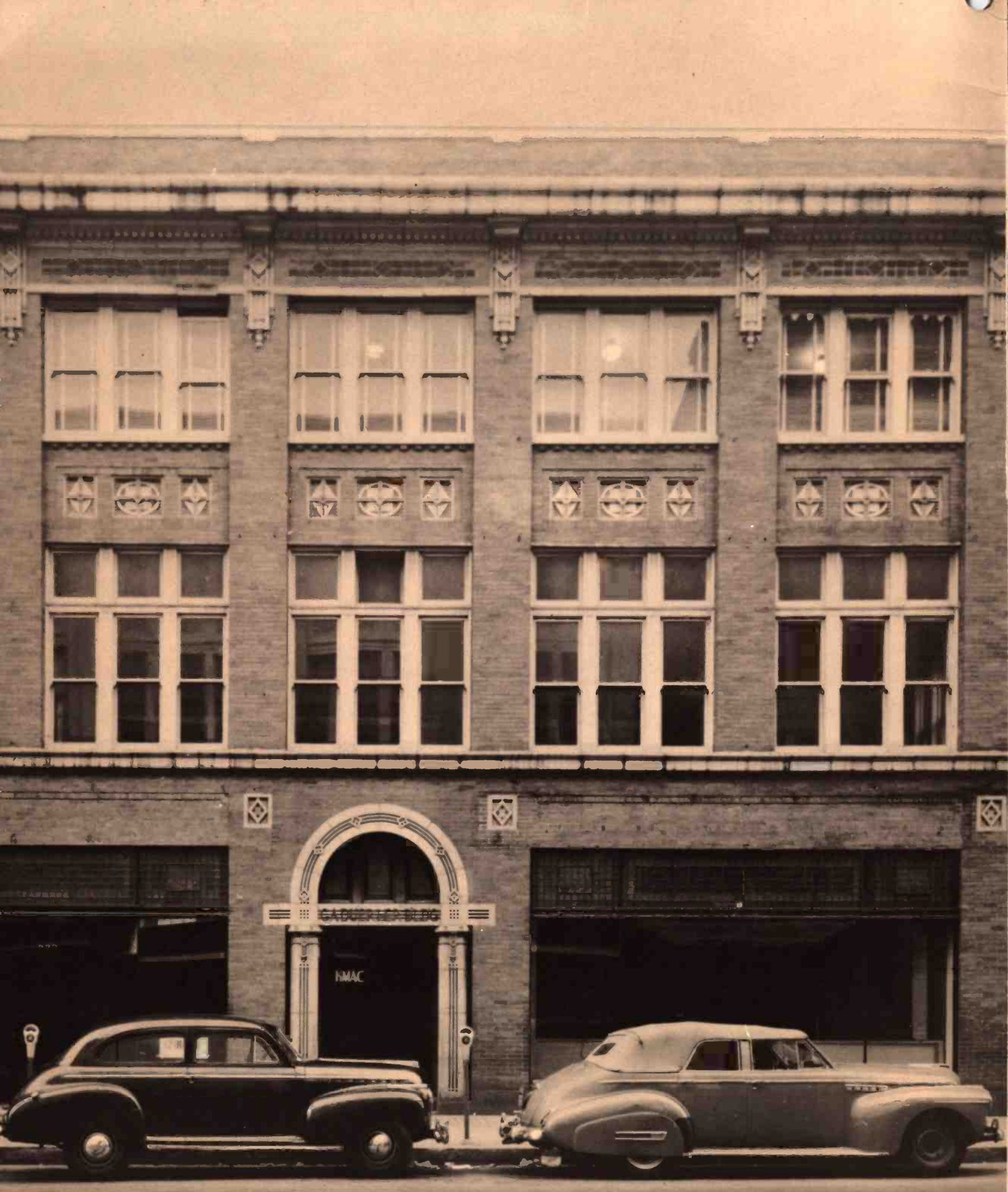
The new home of KMAC-KISS is at 222-24 West Commerce Street
