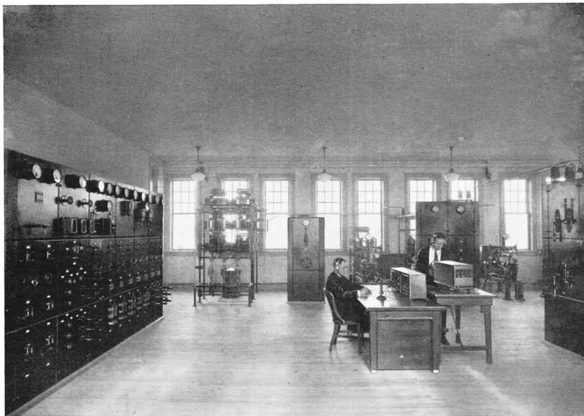
KOA POWER HOUSE ROOM
