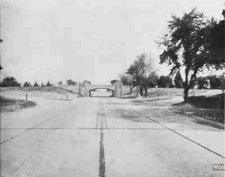
The highway bridge at the intersection of Lindberg and U.S. Highway 66.
