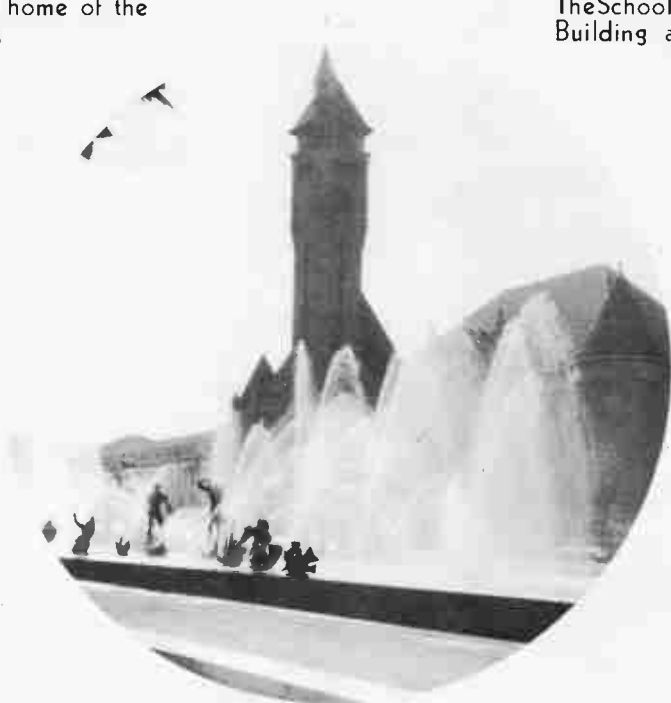
Union Station with Milles Fountain in the foreground.
