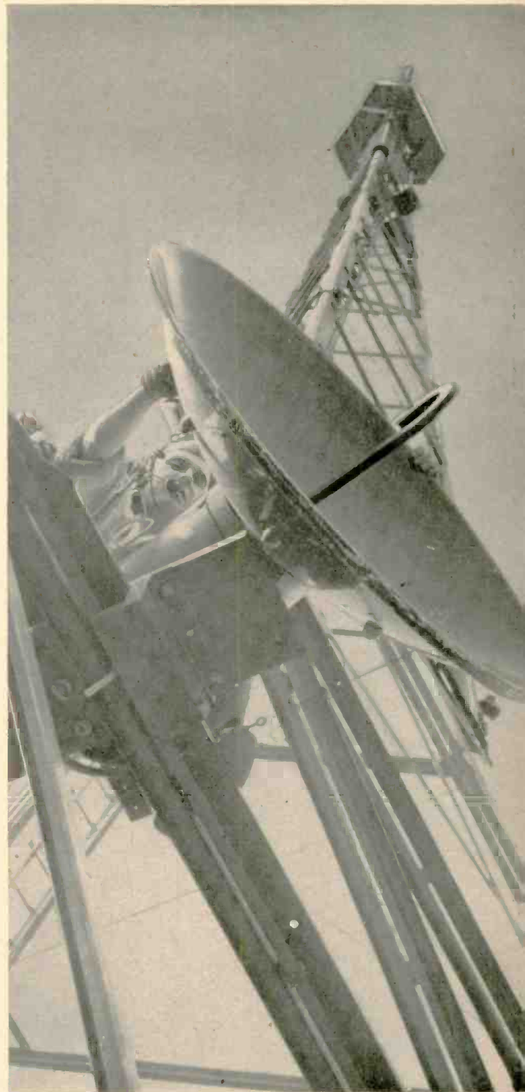
WCAU-TV's relay receiver is located on a high tower in Philadelphia. It facilitates pick-ups from wider areas
