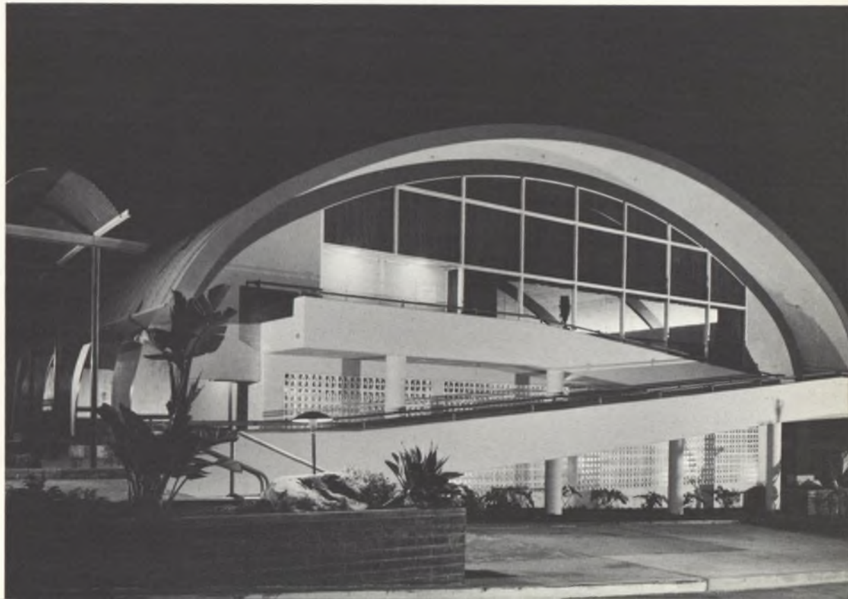
New TV network audience and studio facility—ABC Television Center, Hollywood.
