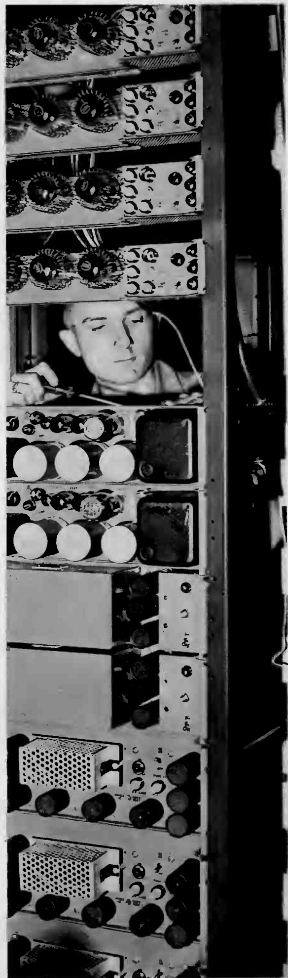
Bill Conrad works on intricate wiring.
