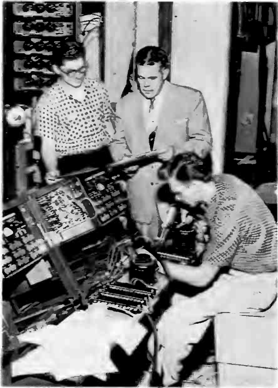
Bill Howard goes over wiring diagram of new studio control board with Dick Ellis as Dave Csik solders.
