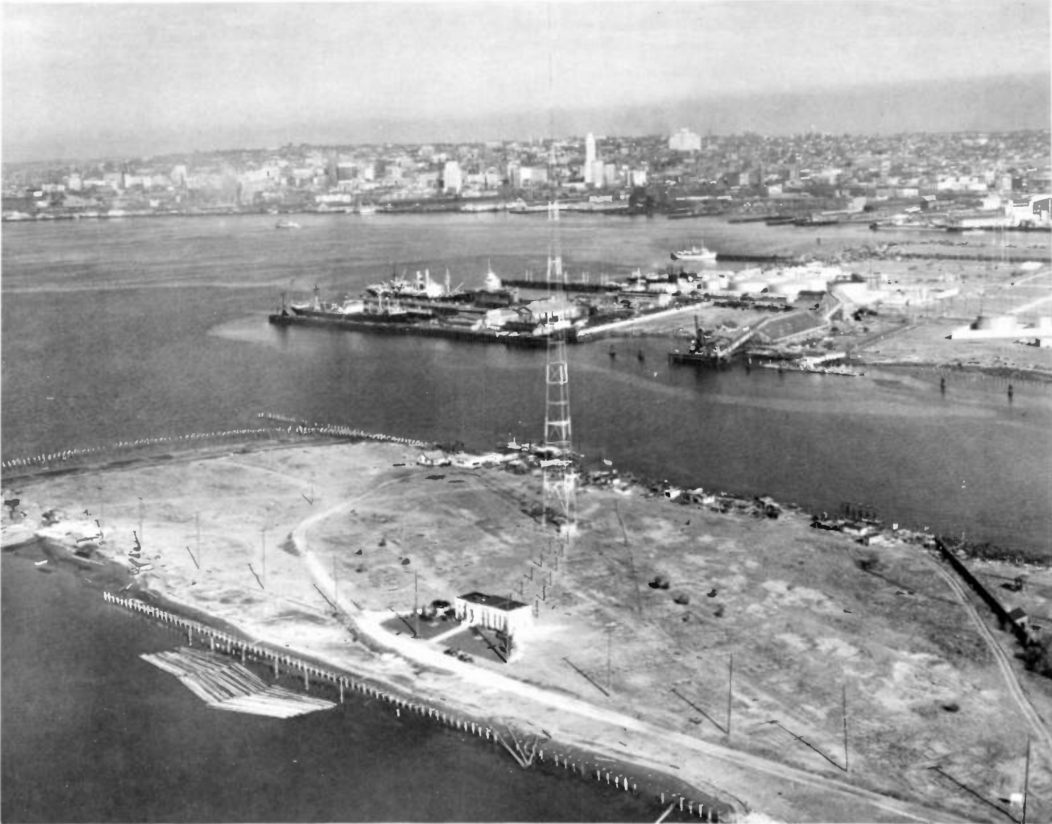
KOMO and KJR shared this transmitter building and 570-foot antenna tower on Seattle's West Waterway after the Fisher company acquired the second station in 1933. The new installation is pictured here shortly after its completion in April, 1936.
