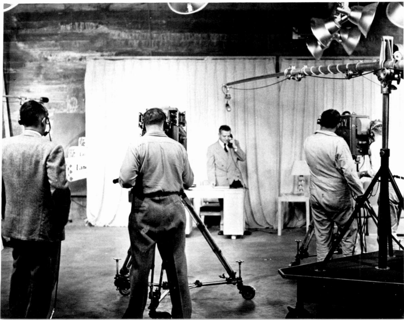
KING-TV studio about 1952. The white desk was used for commercials, besides comprising the “news set” among other things. Note simple traveling-curtain backdrop hiding rough concrete walls. The studio was a converted garage at Second Avenue West and Thomas Street in Seattle.
