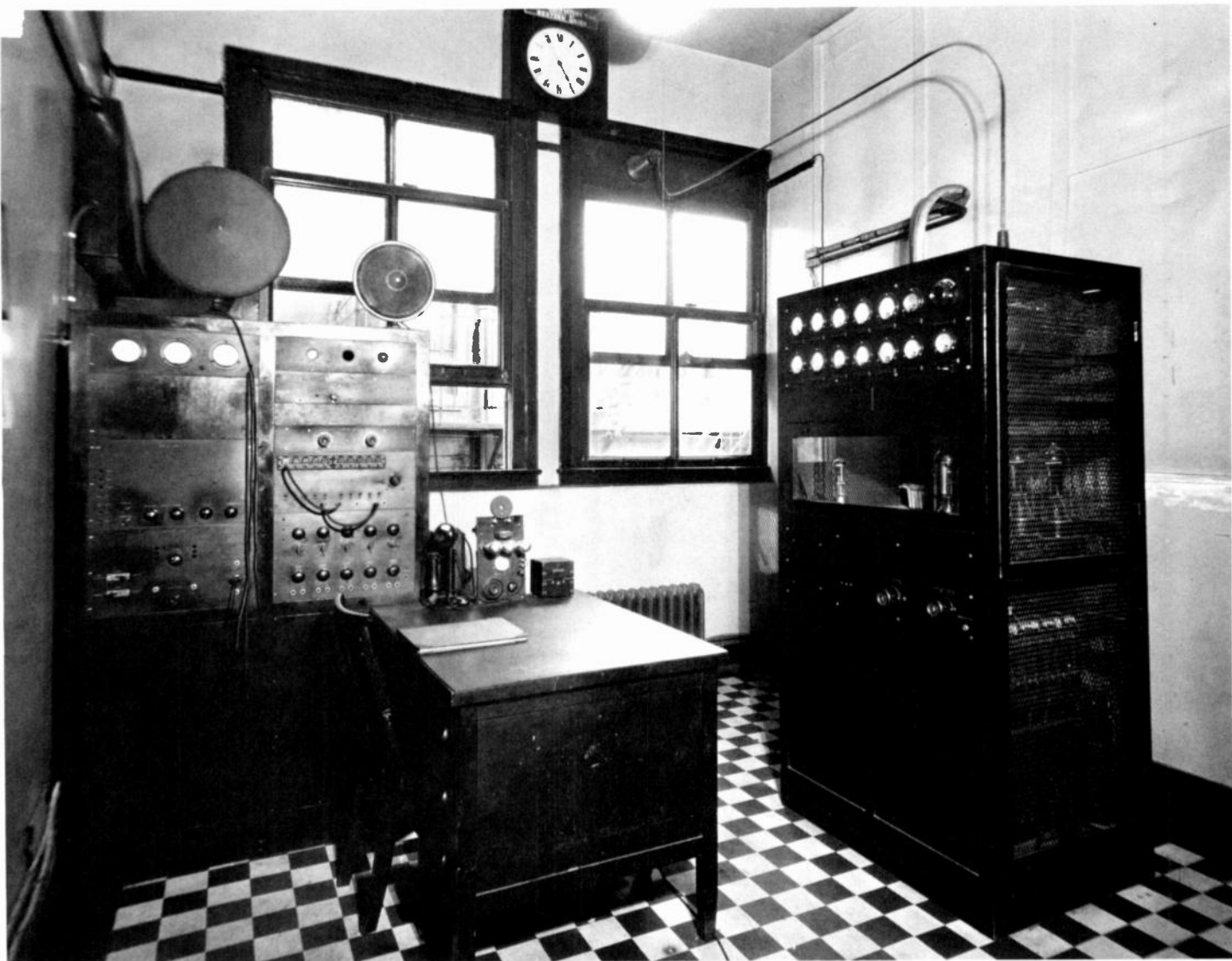
KXA transmitter room, Bigelow Building, in the early 30's.
