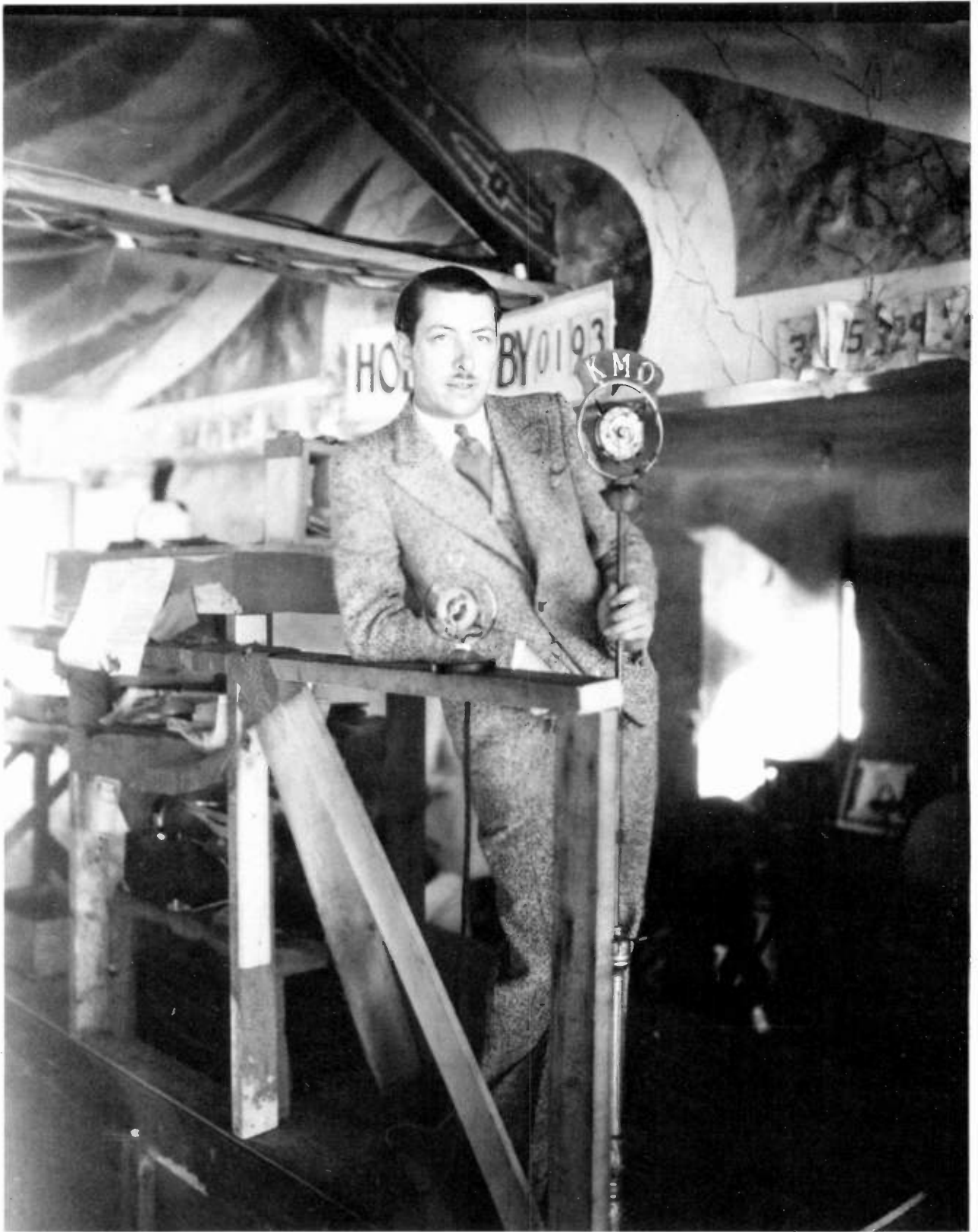
The look of old-time radio. This natty, unidentified impresario is broadcasting by "remote control" from somewhere around Tacoma, about 1930. This may be one of those dance marathon broadcasts that were all the rage. Note that KMO was still using "double-button" carbon microphones.
