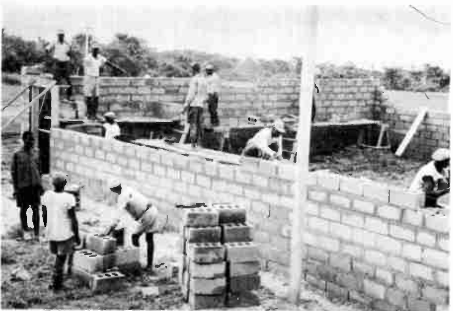
Construction gets underway.
