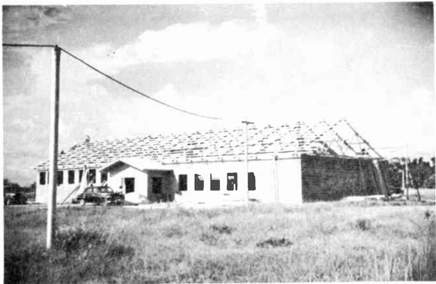
The building takes shape.
