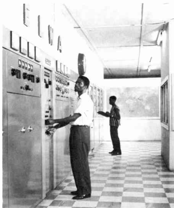
Liberian technical staff reading meters in transmitter building.
