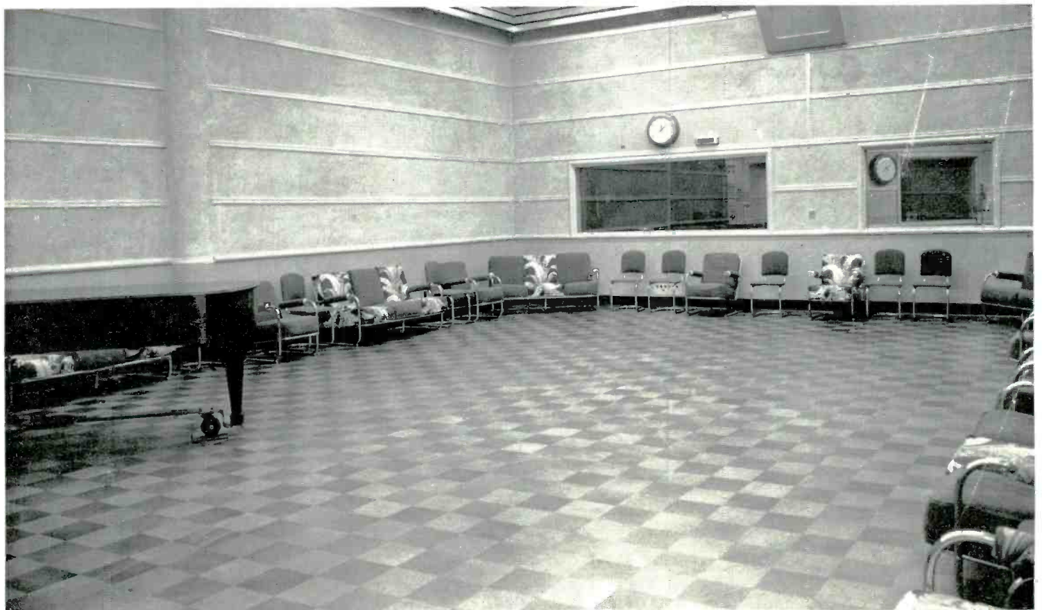
STUDIO A — 21,600 CUBIC FEET LARGEST STUDIO IN WADC'S NEW BUILDING
