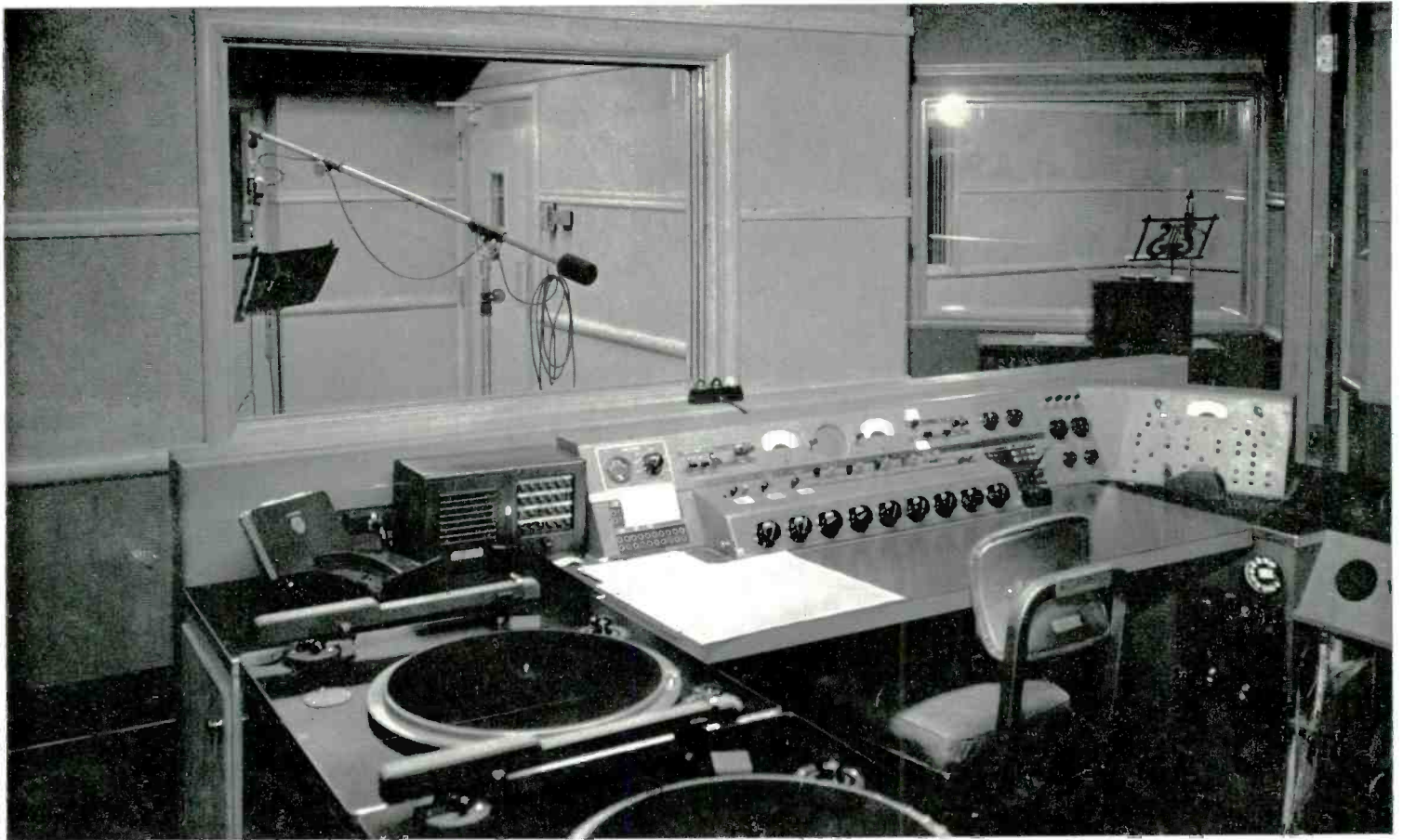
MASTER CONTROL DESK SHOWING SPECIALLY BUILT SWITCHING CONSOLE AND TRANSCRIPTION TURNTABLES IN THE WADC BUILDING NOW.
