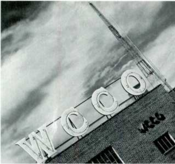
In 1930 construction began on a new WCCO Radio transmitter building which was completed in 1932.
