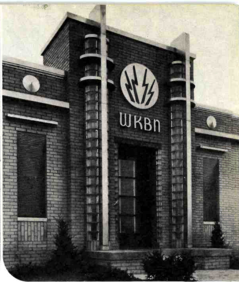
A close-up of the attractive front entrance to the transmitter building, with its cream-colored brick, translucent glass pillars which are illuminated at night, and special effects in stainless steel metal trim.
