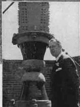
Powel Crosley, Jr., photographed at the base of the 831-ft. antenna of 500,000-watt WLW. The two cup shaped porcelain insulators, with walls less than two inches thick, support a stress load of more than 900,000 pounds.
