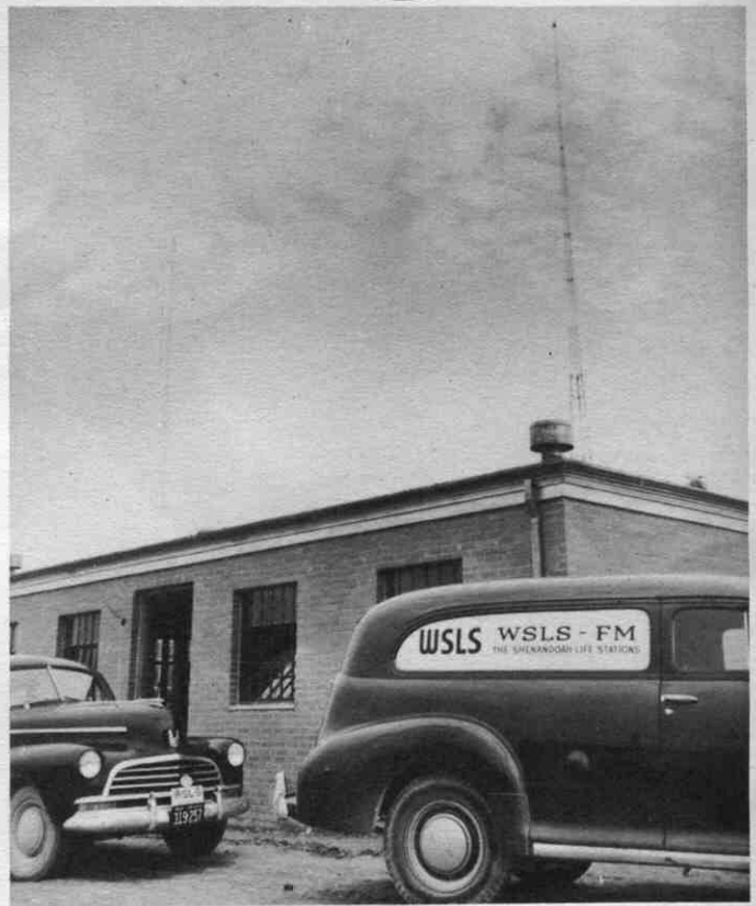
The WLS-AM transmitter site is located between Roanoke and Salem, near Lakeside. Shown here is the transmitter house with two of the four huge 385 foot transmitter towers in the background.
