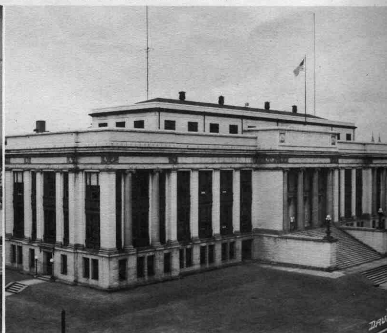
The Roanoke Municipal Building.
