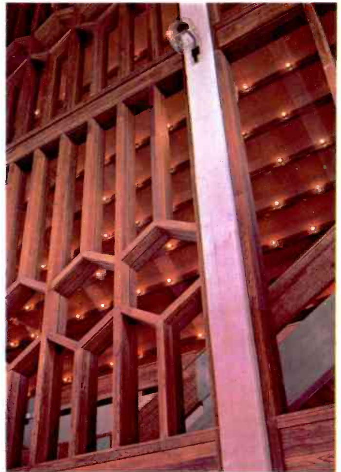
Clear glass set into dark oak frames create a visual relationship between interior and exterior.
