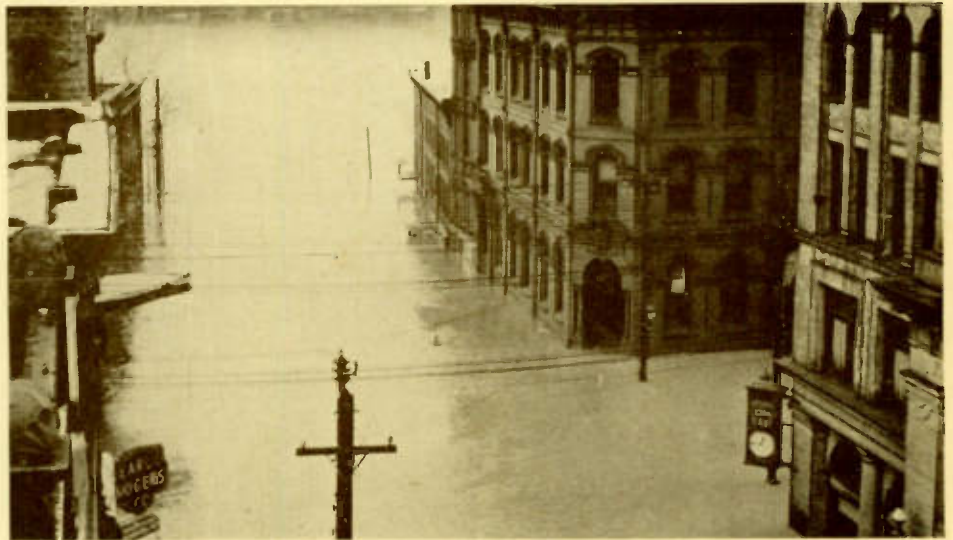
Flood scene at 12th and Main Streets, one of Wheeling's busiest corners. The building dominating the picture is the Hazlett Building and at the left in the foreground can be seen the top of the Earle Rogers Co. building.
