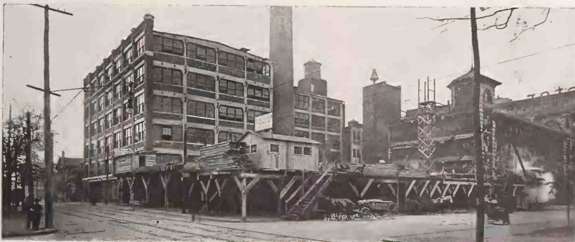
The Pressing Plant Extension to the Victor Co.'s Plant.
