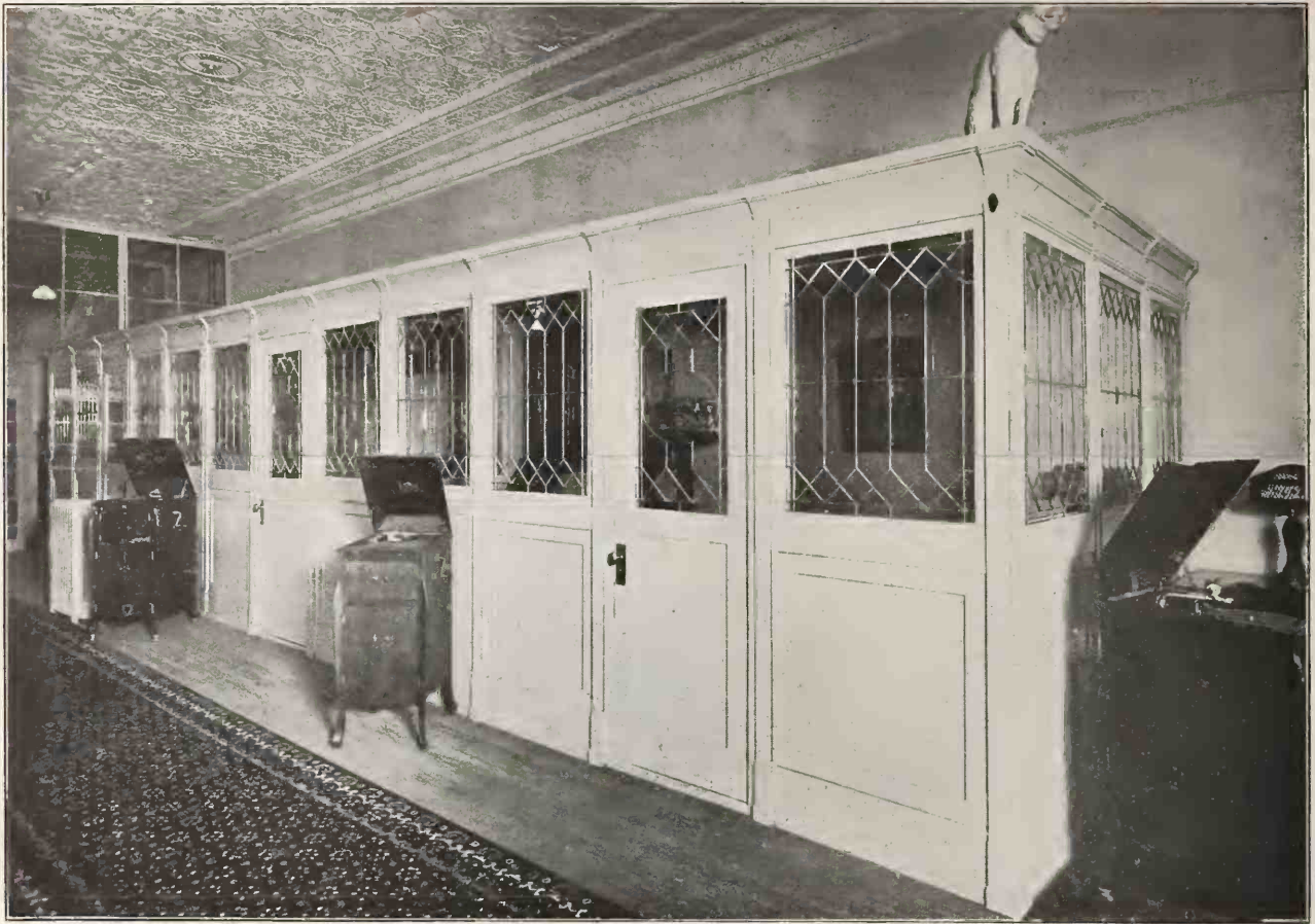
Installation for L. K. Beach Co., Columbus, Ohio
