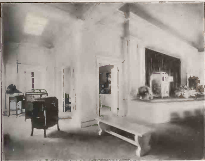
The Stage, Rest Room and One of the Demonstrating Booths.
