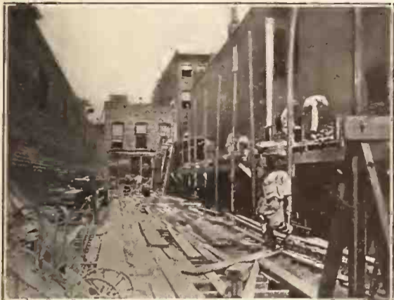
Starting Work on Corley Building
