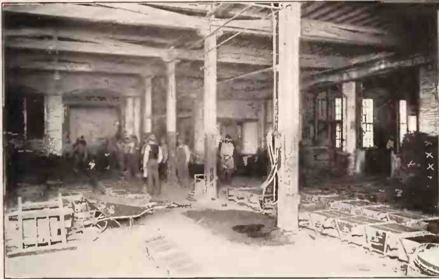
5. Foundry (Another View)
