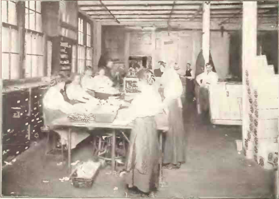
27. A Corner of the Packing Room
