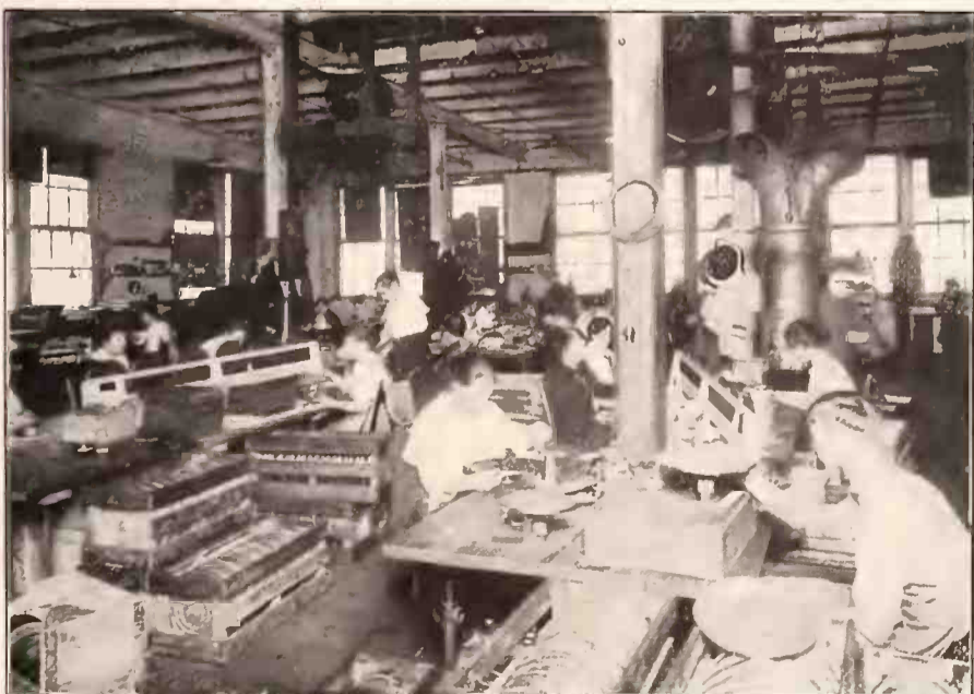
24. Turntable Covering and Testing
