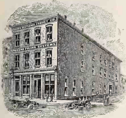
The New Ogden Plant
