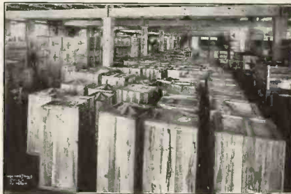
One of the Vitanola Storage Rooms
