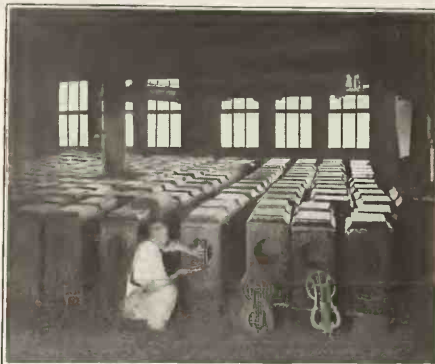
Part of Finishing Plant
