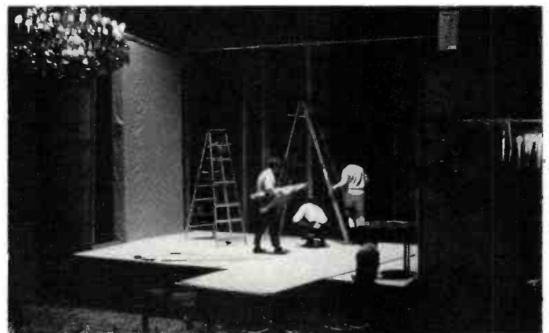
Carpenters (above) erect stage at Plaza. RKO General planning team of (l. to r.) Joe Cook, Al Korn, Mort Zimmerman, Lionel Furst, Don Quinn and Jack Duffield get together at rehearsal hall for strategy meeting.
