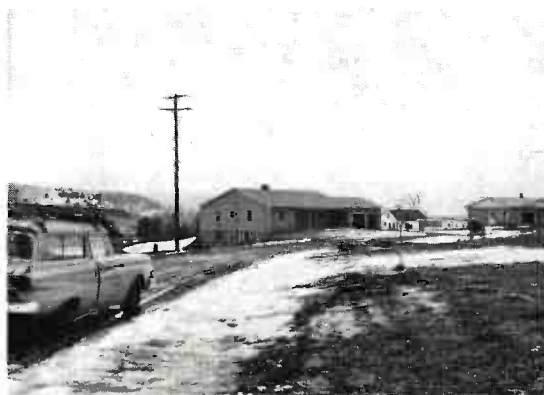
The Coes extended their cable run last year to 17 homes in this new housing development.
