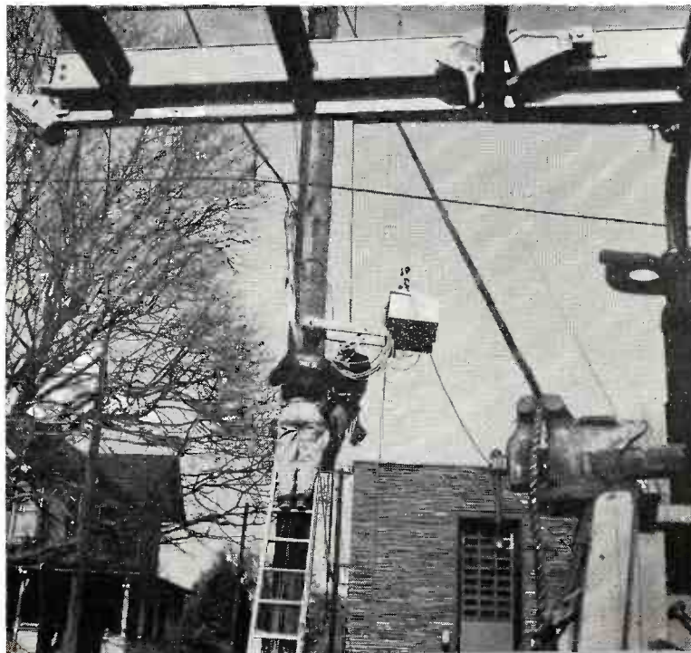
Auxiliary antennas sprout on system's tower equipment building. Repair crew switches amplifier from old to new telephone pole.
