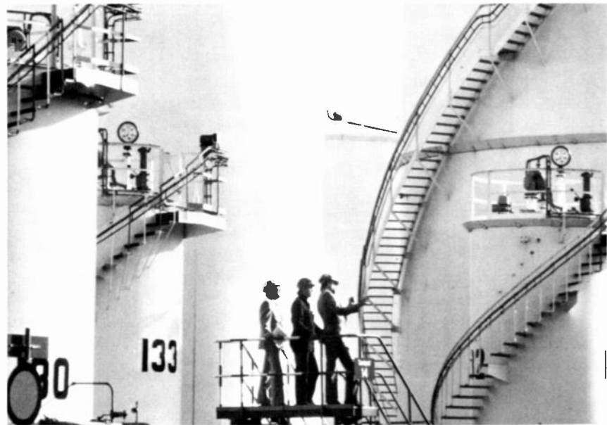
Figure 1. ( Computer: Impact—Impact on the Work Force ) At a refinery in Rotterdam, ST 3000 smart transmitters accurately measure and control process flow, liquid level, and pressure. Courtesy of Honeywell, Inc.
