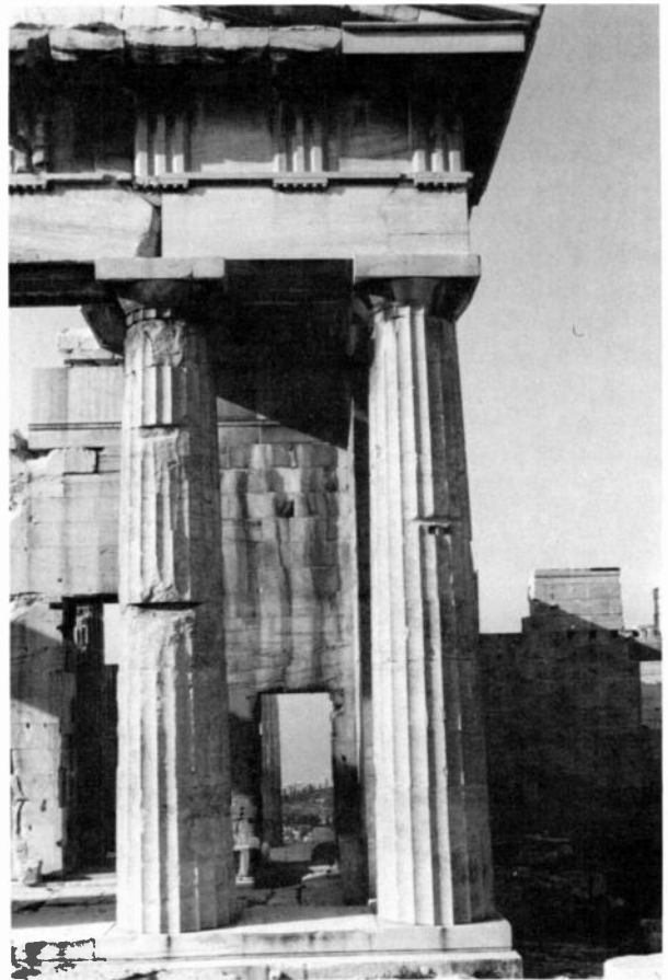
Figure 1. (Architecture) The Doric order. The Propylaea, Athens, 437 B.C.E. Courtesy of Christian Norberg-Schulz.
