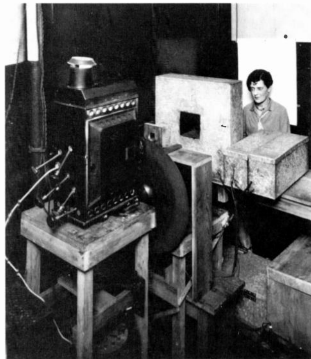
Figure 2. ( Television History—Early Period ) Scanner with Nipkow disk, as used by General Electric in experiments in the 1920s. Smithsonian Institution, Washington, D.C. Photo No. 60,005.
