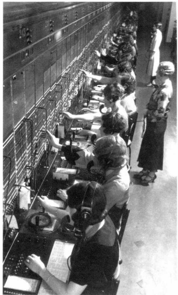
Figure 2. ( Telephone ) Early telephone switchboard. The Bettmann Archive, Inc.
