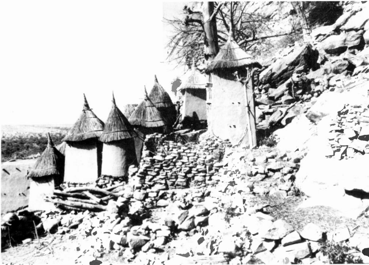
Figure 10. ( Africa, Precolonial ) View of traditional house architectural style and building materials in the Dogon village of Sangha, Mali, 1971. United Nations photo 120924/J. Laure/PAS.
