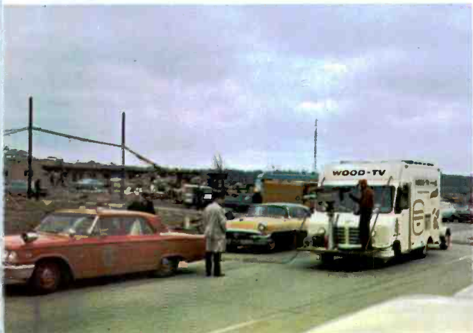
WOOD-TV's remote unit on the scene at 1965's tornado damage.
