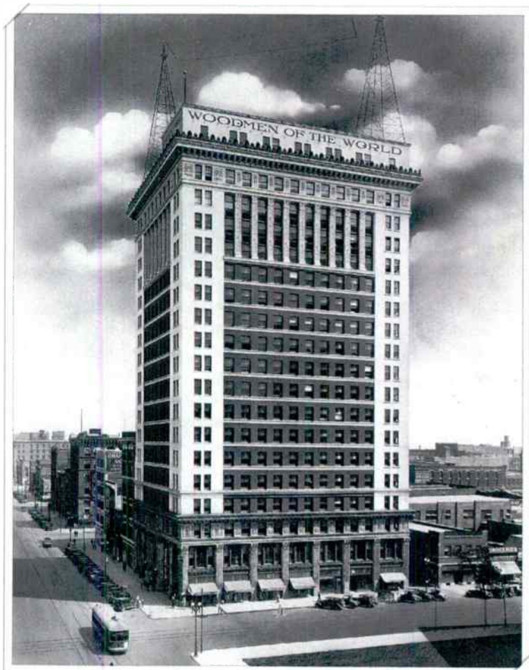
Woodmen of the World Building with the WOAW rooftop 19 th story addition and towers on top of the building. (WOW Archives)
