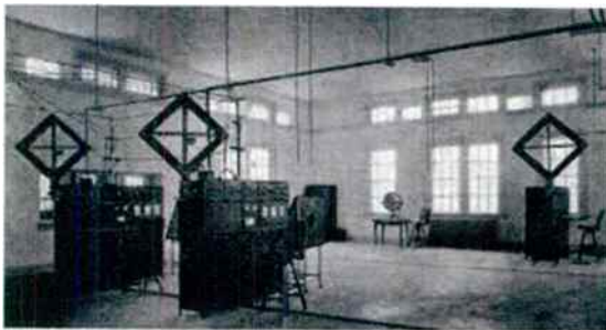
Some receiver work consoles in the Grand Island Monitoring station with rotatable loop antennas used for direction-finding.
