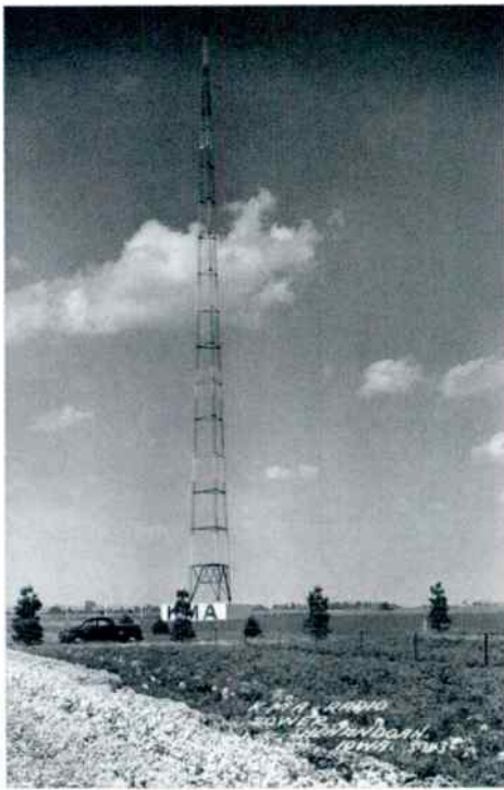
KMA's new tower, replacing the flat-top antennas at the seed company.
