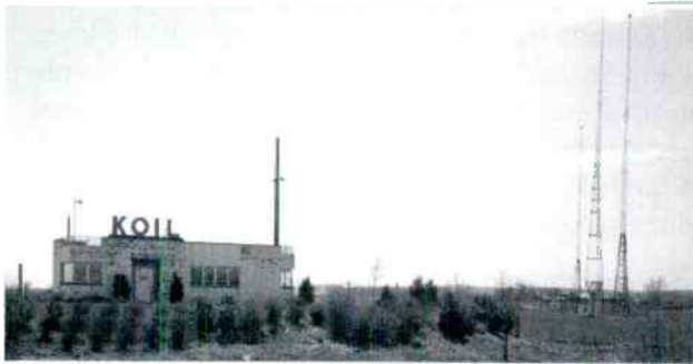
KOIL's Manawa transmitter site with its new three-tower directional tower system (1943 photo. © Durham Museum)
