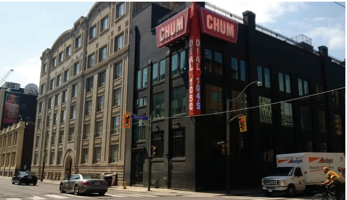
The Bell Media broadcast complex in downtown Toronto has a 299 Queen Street West address but it embraces other buildings on the block, including the historic building at 260 Richmond, an old (c. 1915) warehouse once owned by Tip Top Tailors.
