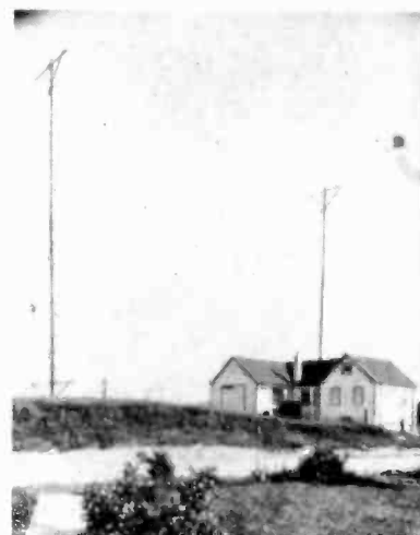
This is CFRB's original transmitter house, a small wooden hut at Aurora, with a single strand of copper wire slung between wooden poles acting as an antenna.
