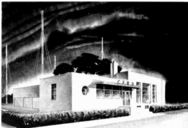
Here is CFRB's architecturally modern yellow-brick transmitter house on the Lake Shore Highway. Floodlit at night, the layout will soon be enhanced by landscape gardening and the addition of a brilliant neon sign.
