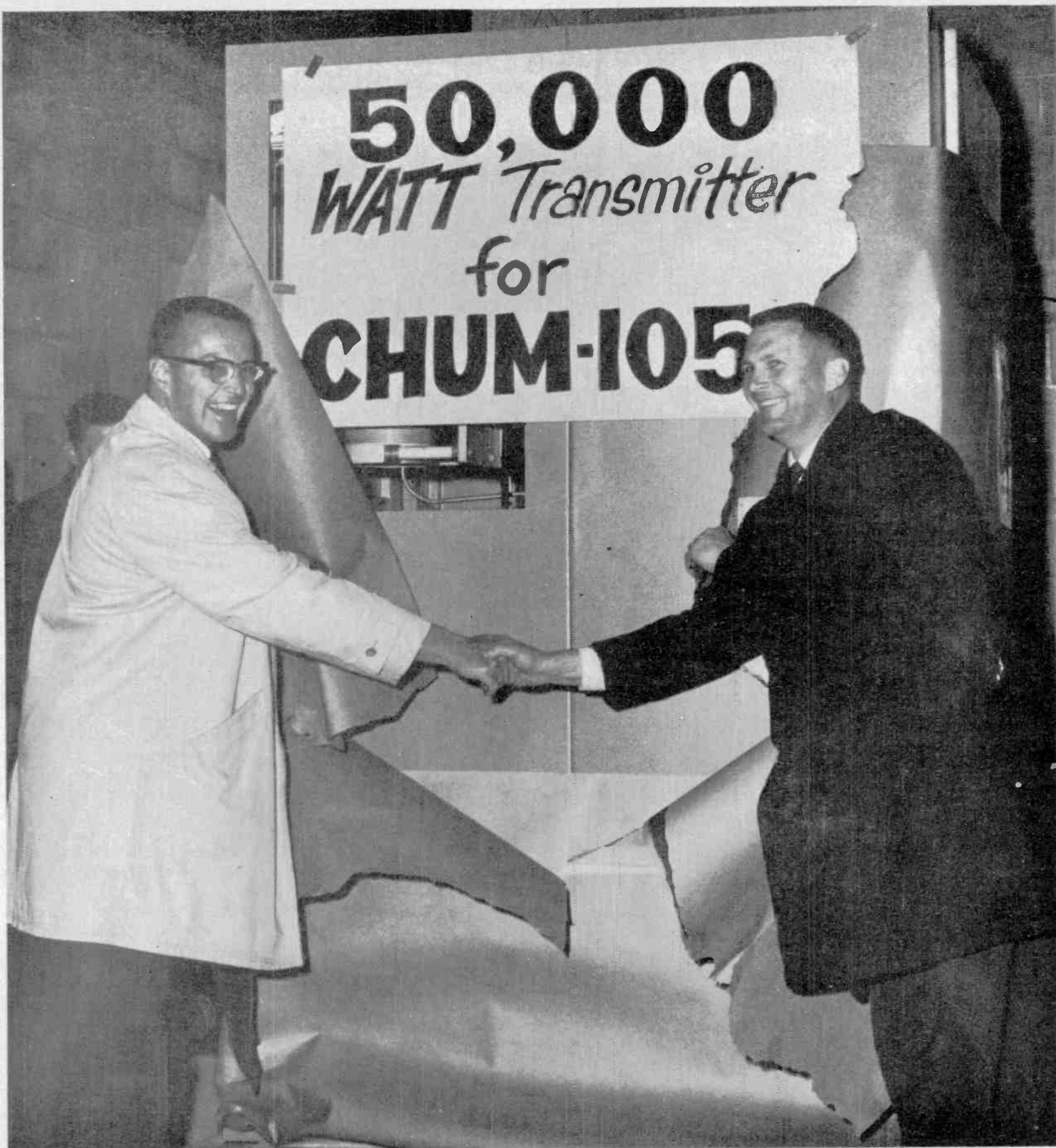
CHUM President, Allan F. Waters (left) and Chief Engineer, George Jones, accept delivery of CHUM's long-awaited 50 kw transmitter // It took 12 men to move the valuable cargo from the truck to the main transmitter building on the property of the CHUM-owned Rockway Motel, Highway 2 near Clarkson // The six transmitting towers are up, construction of the six individual tower buildings is completed, and construction of the main transmitter building is nearing completion // CHUM-1050... soon 50,000 watts
